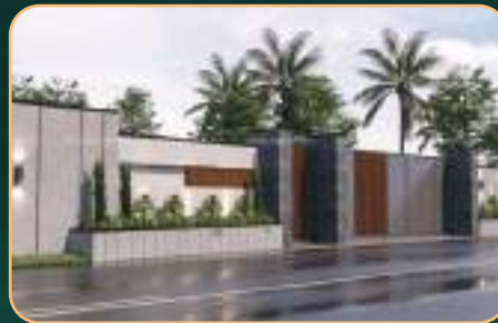
BOUNDARY WALLS FOR PRIVACY
