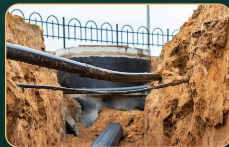
UNDERGROUND ELECTRICITY & SEWERAGE
